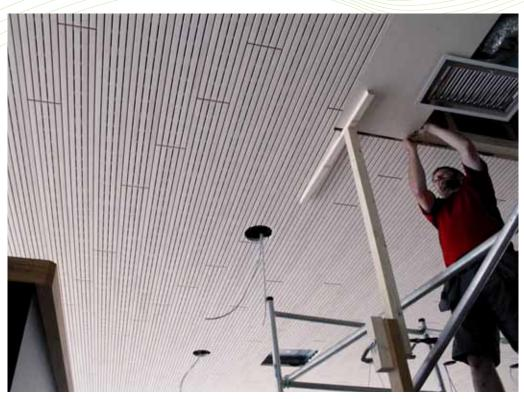
Thanks to the compact form of all components, the lenofon soundproofing panels can be easily placed even by a single fitter.
