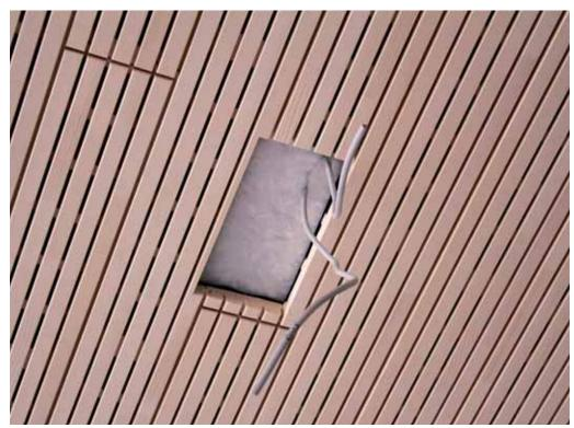
To install any flush-mounted fittings (e.g. lamps, speakers etc), cut the placed panels with an electric fret saw or a hole saw.
