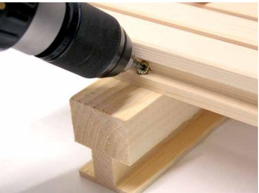
Simple installation of the support structure, of the insulation layer and of the lenofon panels.
