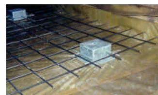
The boxes with reinforcement
