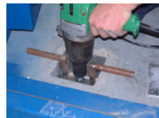
Jacking up the slab
