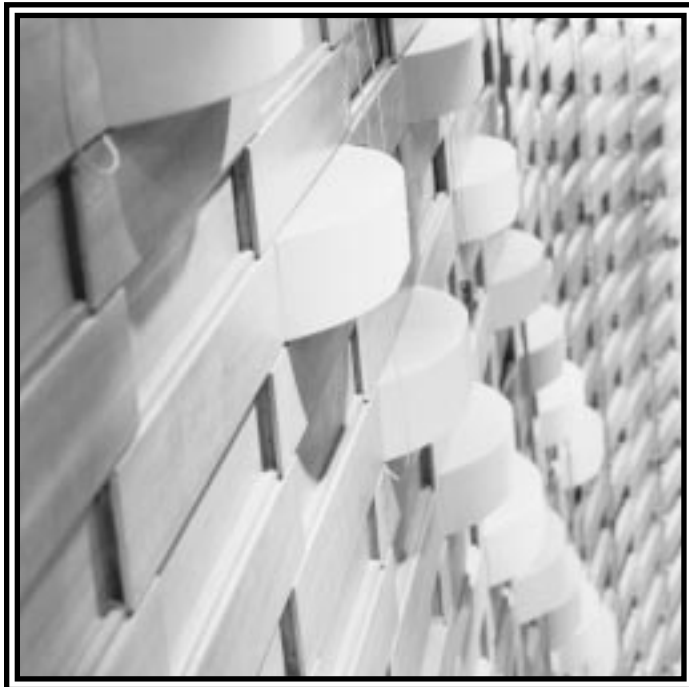
Close-up of optimized diffusers in basket-weave curving wall
