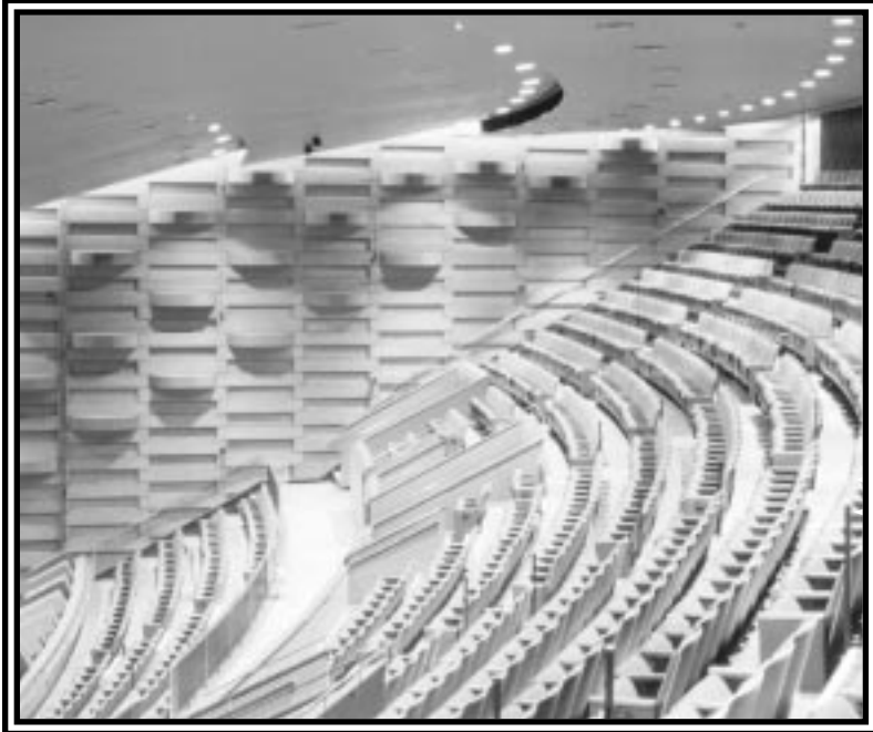
Overall view of side wall integrated diffusers, audience seating and ceiling.
