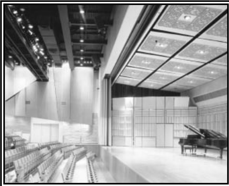
Closeup view of the rollable side VAMPS® towers and side wall of the auditorium.
