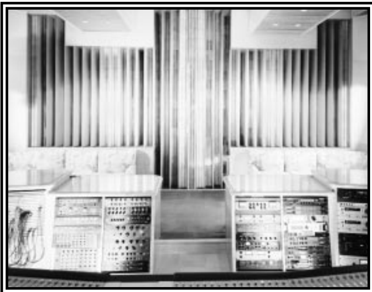
Gallery Control Room Diffusion Wall with custom ceramic Diffractal® elements
