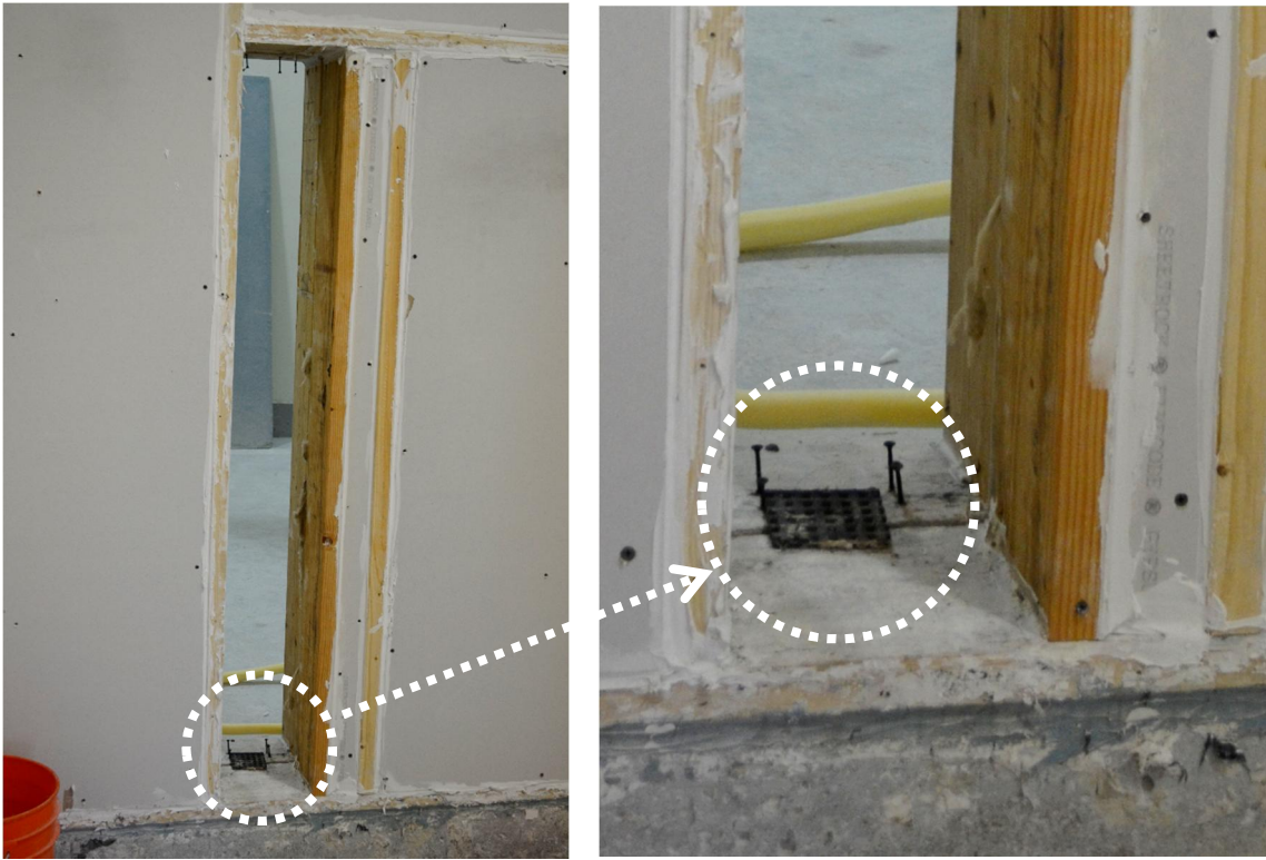
FIGURE 4-4: IMAGE OF HOLLOW EXPOSED MULLION PROFILE WITH ANTI-BUCKLING CLIPS, WOOD SPACES AND SILICONE GASKET
