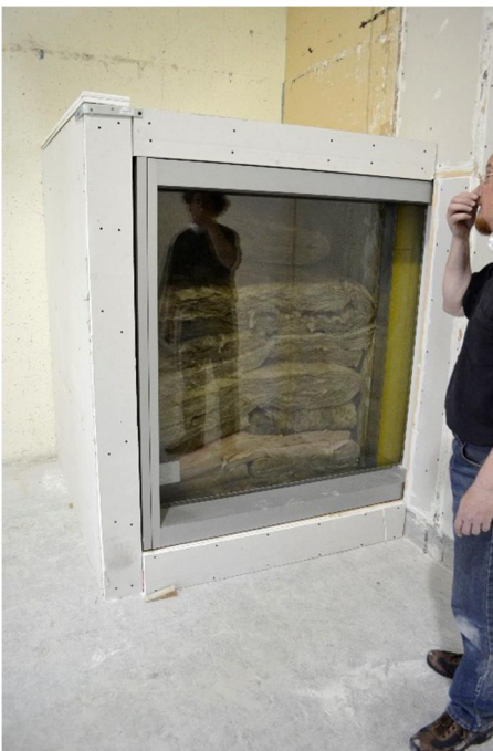
FIGURE 4-65: CHAMBER 3S (BUILT WITHIN THE WEAL SOURCE CHAMBER)
