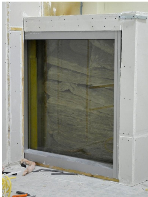
FIGURE 4-66: CHAMBER 3R (BUILT WITHIN THE WEAL RECEIVING CHAMBER)
