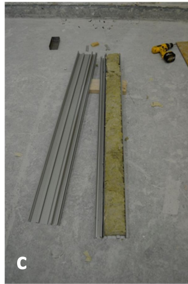
FIGURE 4-12: CLASS B FILLED MULLION (A) PEA GRAVEL (B) SAND (C) MINERAL WOOL (D) MLV PILLOWS
