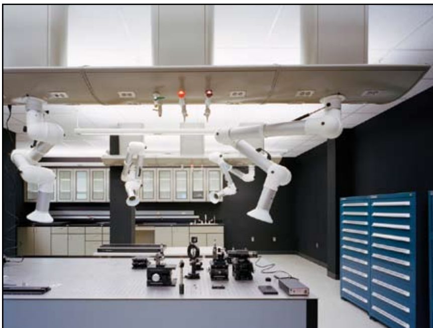
Vibration table used to place vibration sensitive equipment; Rochester Institute of Technology.
