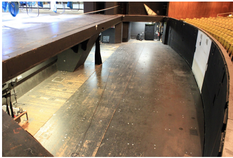
Figure 5. The orchestra pit at Deutsche Oper Berlin with the overhang below the stage (left).
