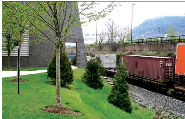
Figure 1. USX rail line adjacent to UPMC Sports Medicine Center building.
