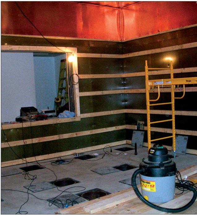
Figure 12. Vibration isolated MRI room during construction.
