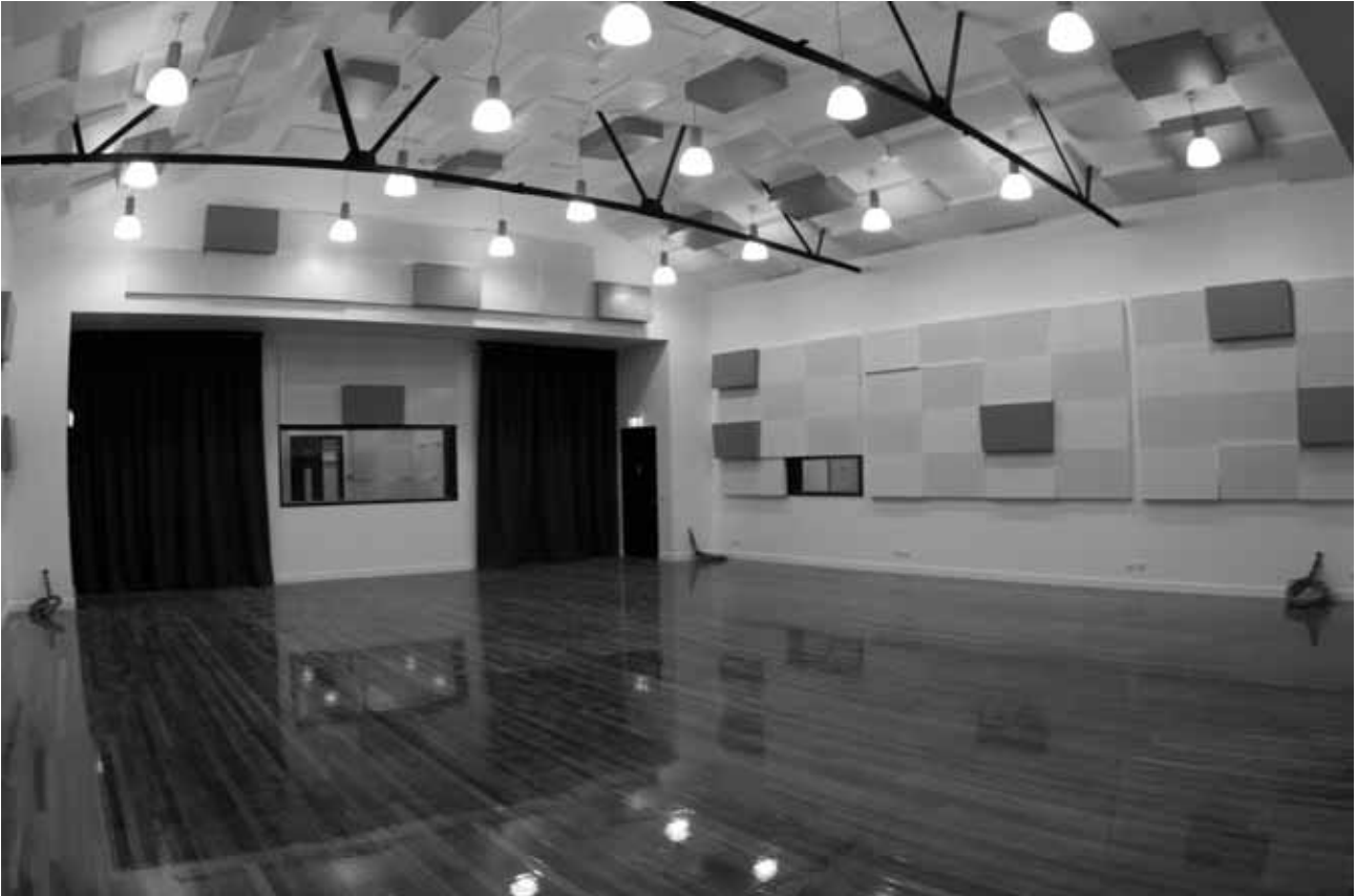
Figure 6: Main studio nearing completion.
