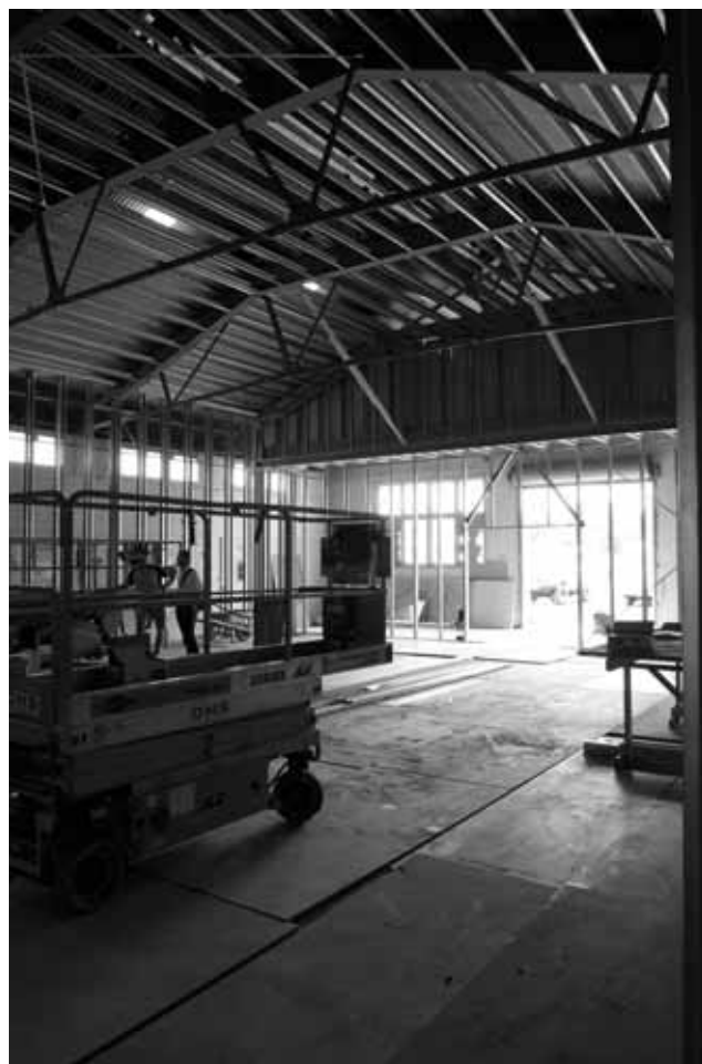
Figure 3: Studios under construction.
