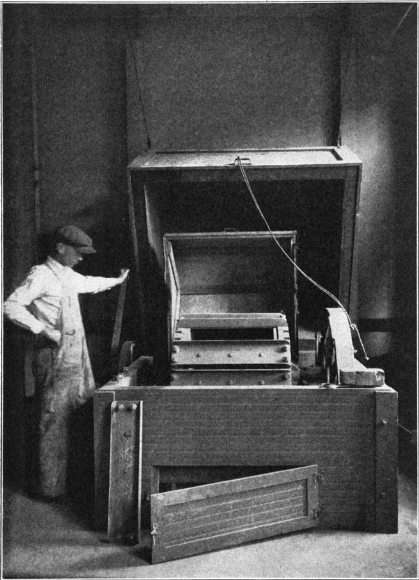
FIG. 30. SOUND-PROOF BOX TO REDUCE NOISE OF BRICK RATTLER
