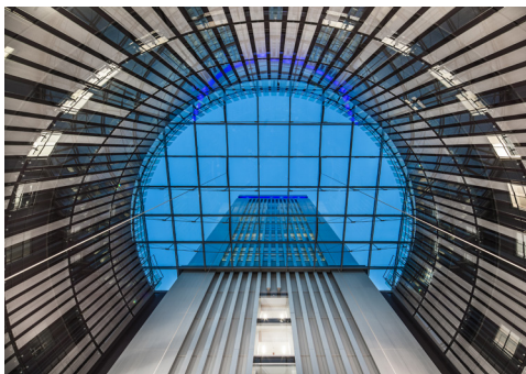
The tower, seen from the Agora
