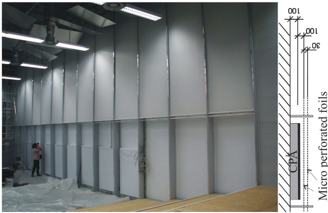
Figure 1: CPA and micro-perforated foils on the side walls of the rehearsal room of the Staatstheater Stuttgart.
