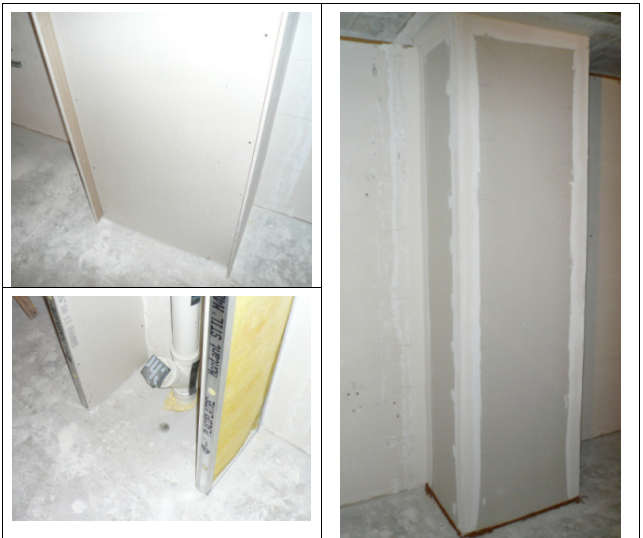
Gaine N= 1 : Cloison Placostil® 72/48 – BA13 Std
