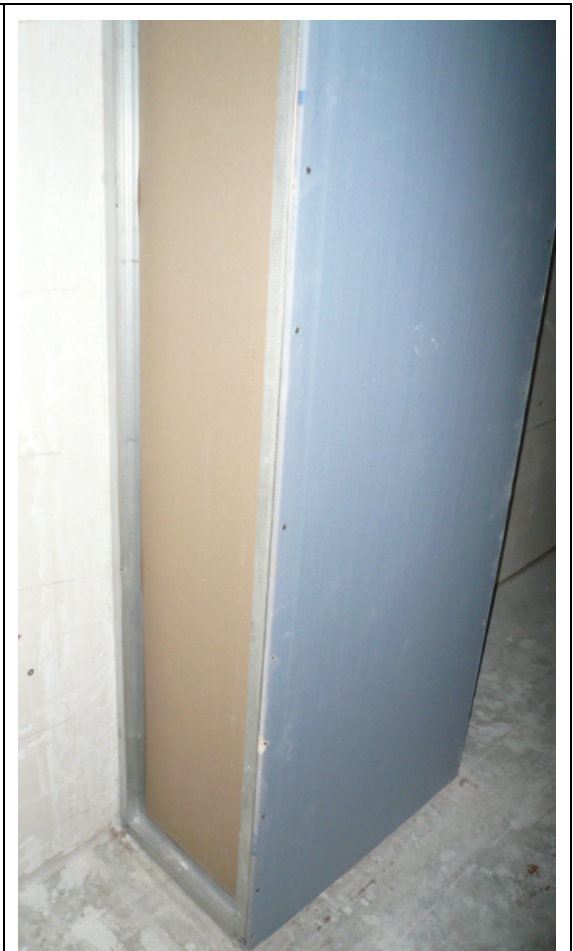
Gaine N= 2 : Cloison Placostil® 72/48 – BA13 PPH
