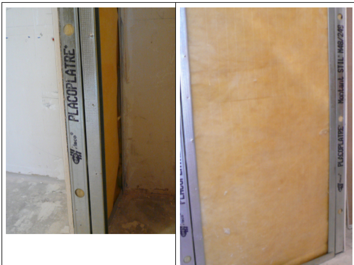
Gaine N= 2 : Contre-cloison Placostil® 72/48 – BA13 PPH
