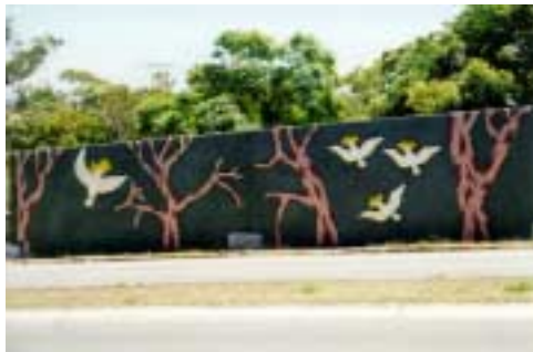
Figure 4.3 A 160° subtended angle at a reception point is generally considered to provide a minimum barrier length. If this barrier attenuated noise by 11 dB(A), an “infinite” barrier (180°) would provide an attenuation of about 16 dB(A).
