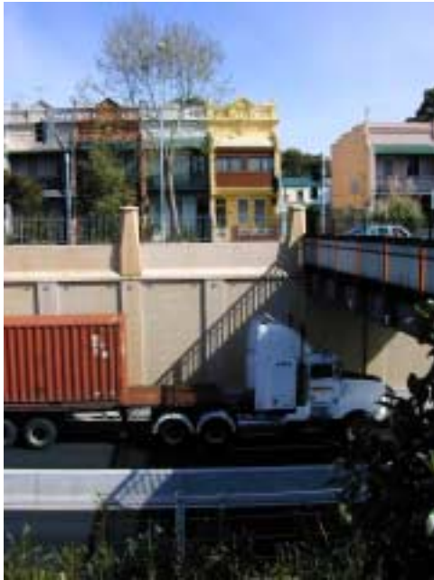
The “sunken” vertical alignment of the Eastern Distributor parkway helps to reduce noise levels at nearby residences
