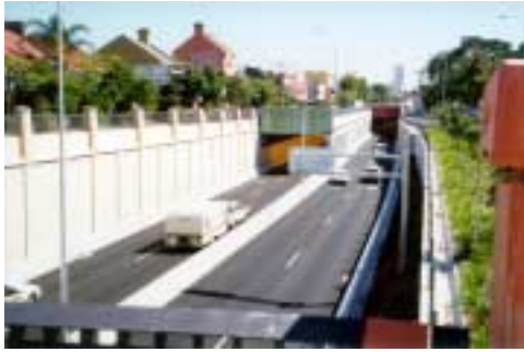
The “sunken” vertical alignment of the Eastern Distributor parkway helps to reduce noise levels at nearby residences
